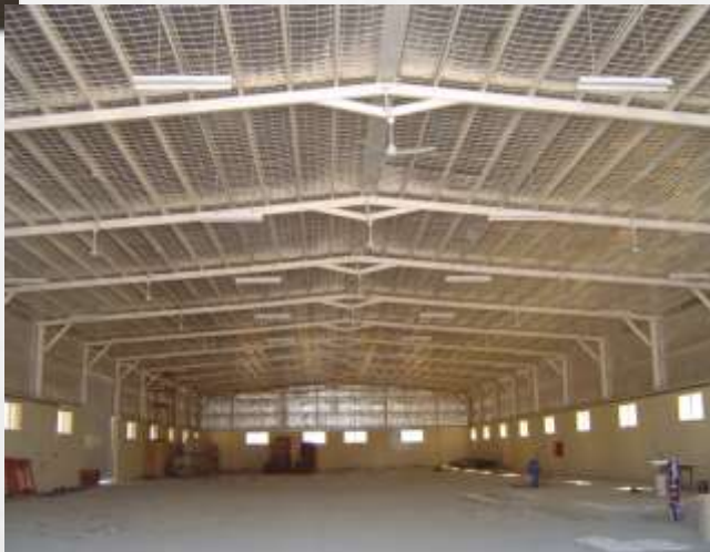
Factory Dubai for Insulation & Technical Industry
