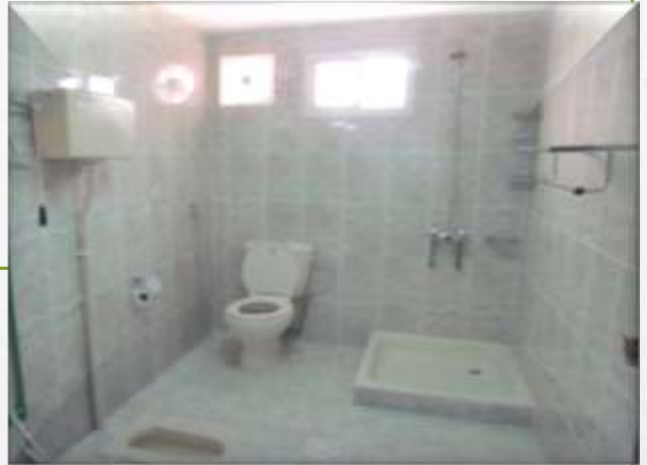
Ablution inside the villa for private customer
