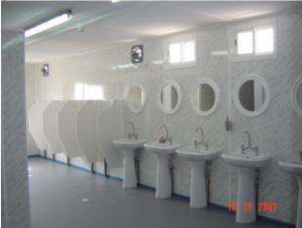
Ablution block for Qatar Kentz at Raslaffan
