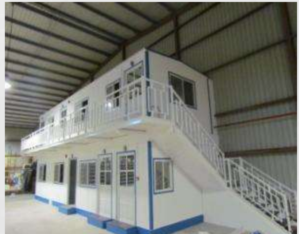
Double Storey Site Office for Oryx GTL at RLIC
