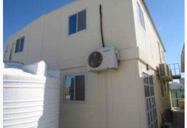
Site office for Dar Al Rokham at Heart of Doha
